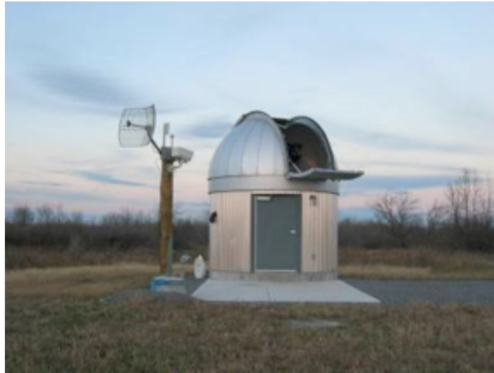
Figure 1: The DRDC SSO as seen from outside. The dome is pictured in its fully open position, with the mast that holds the wireless link antenna, the weather sensor, and the GPS antenna.
