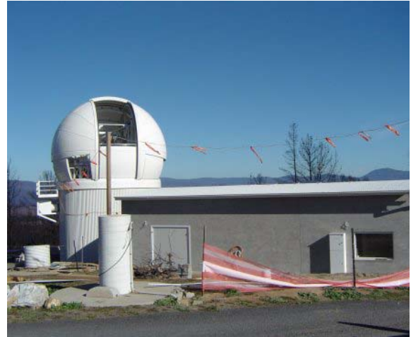
Fig 7. Laser and Control Room Construction
