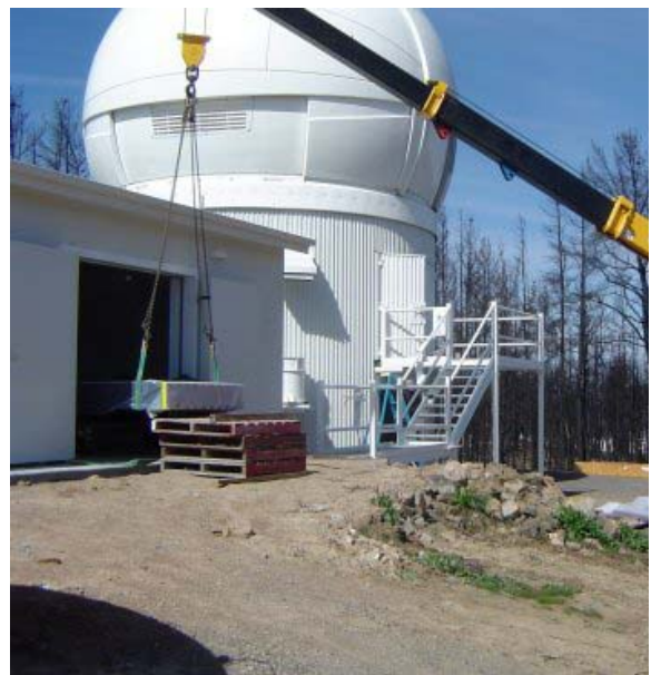
Fig 9. Installation of Laser Tables
