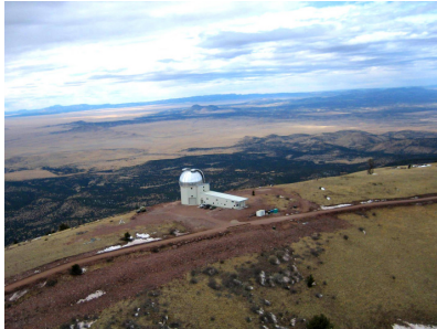
Fig. 1. The Magdalena Ridge Observatory 2.4-meter fast-tracking telescope and support facility located outside of Socorro, NM on Magdalena Ridge. The observatory performs target-of-opportunity scientific research focusing on asteroids and comets along with work in the area of space situational awareness.
