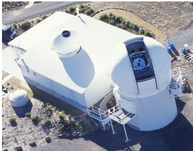
Fig 1: 1.8m telescope with co-rotating observing floor
