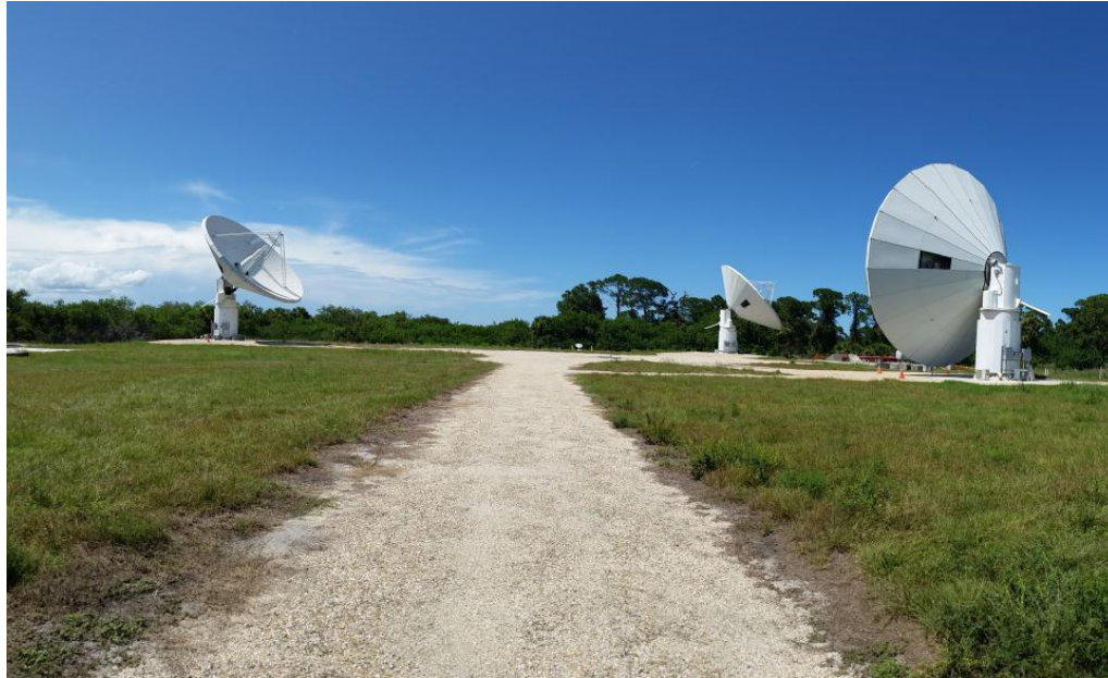
Fig 9. Current Array Configuration of Three 12m Reflector Antennas at the Kennedy Space Center
