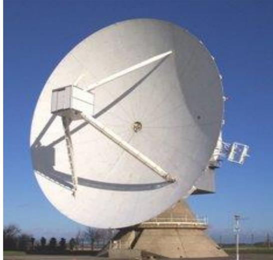
Fig. 2. The 25 m diameter fully-steerable dish
