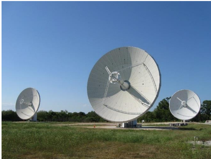
Fig 5. Current array configuration of three 12m reflector antennas at the Kennedy Space Center
