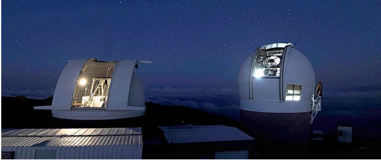
Figure 1: The Pan-STARRS Observatories, located near the summit of Haleakala on the site of what was the LURE Observatory. The PS1 and PS2 domes are precisely north-south of each other, connected by a common support building. Pan-STARRS1 or PS1 (F51) is on the right. The Pan-STARRS2 telescope, or PS2 (F52) is on the left. The optics of both systems are nearly identical. However the telescopes and domes are quite different and were built by different manufacturers. The two observatories are not completely independent — they share power, cooling, computing resources and network connectivity.
