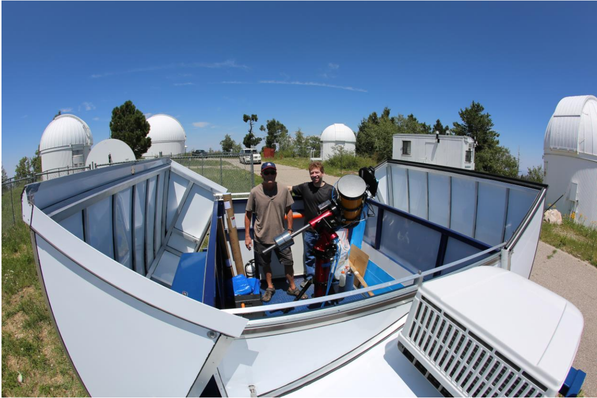
Figure 5. The Dog House in its open position showing the Takahashi E-180 Astrograph. The air conditioning unit can be seen in the foreground.
