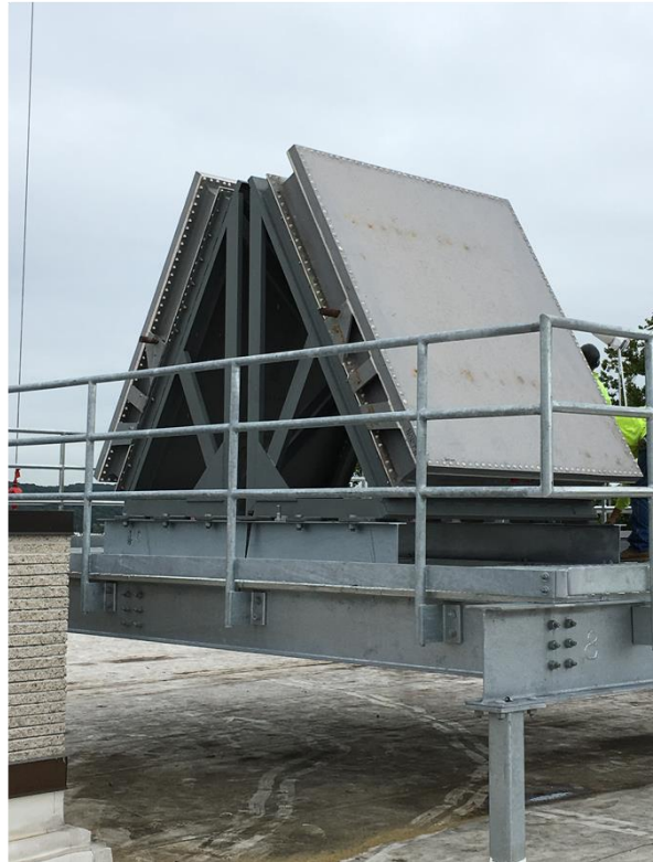
Figure 1: Phased Array Antenna
