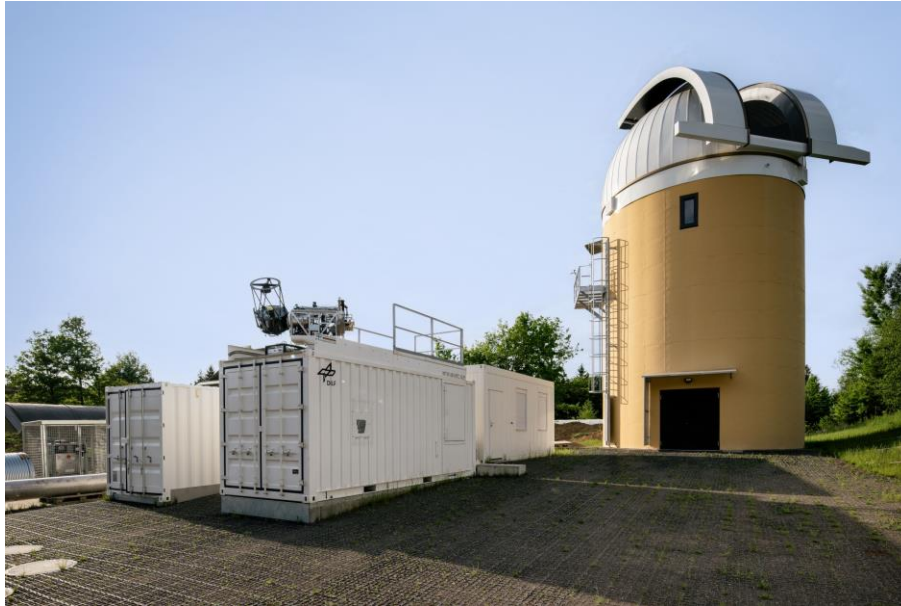
Fig. 2. Transportable station STAR-C (container with elevated telescope mount platform, left) and ground-station JKO (building with dome, right).
